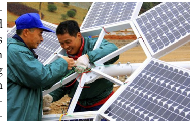
INSTALLING A SOLAR SET-UP IN CHINA
