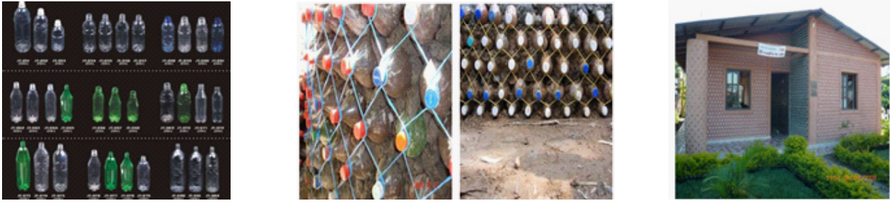
Fig 7. Wall made up of PET bottles
