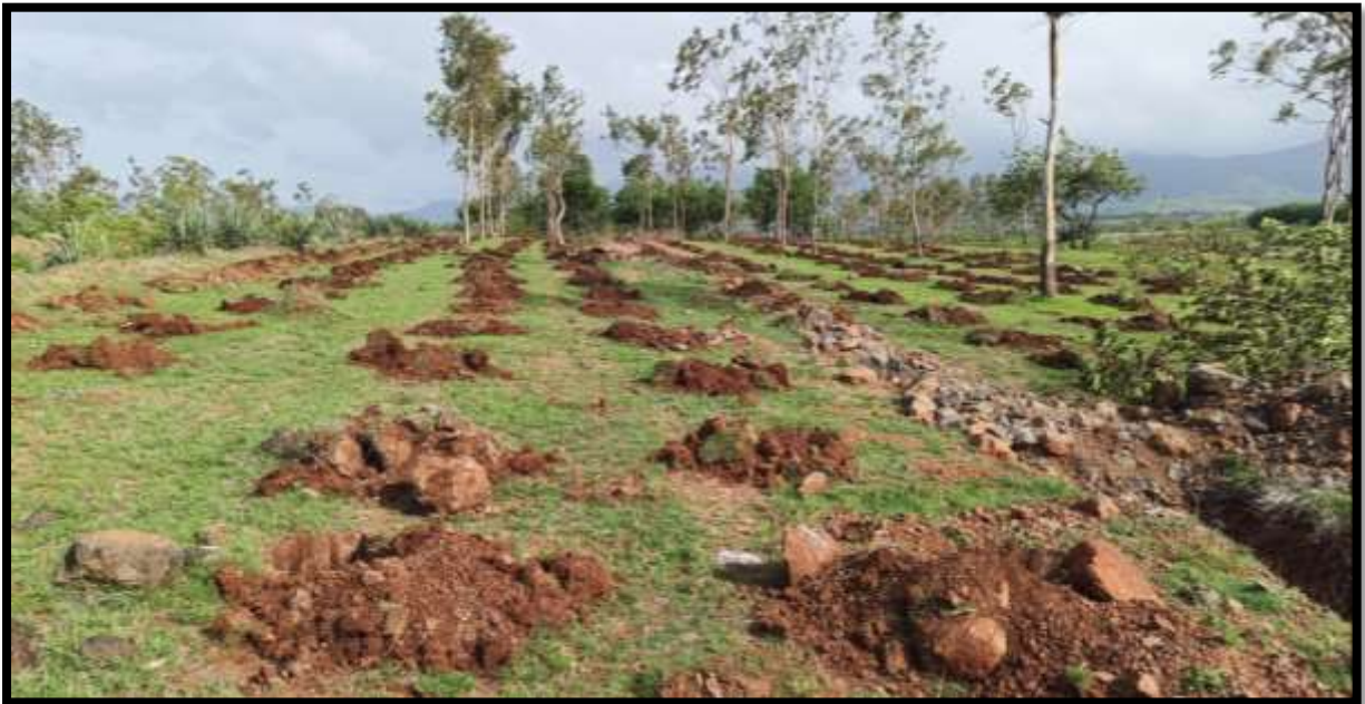
IMG: Site after pits digging completion
